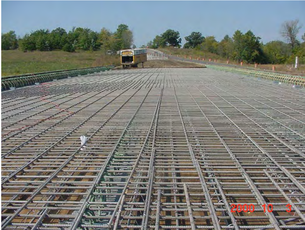
Figure 1. Stainless Steel Reinforcement of Bridge A6059
