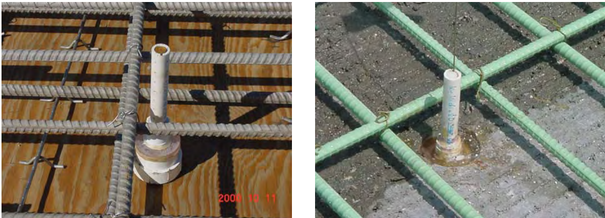
Figure 2. Sensor Housings Installation
