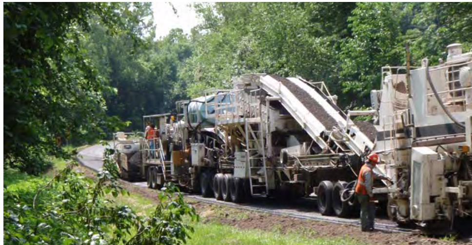
Figure 1 – Paving train
