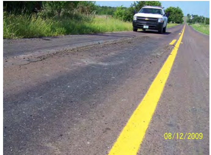
Figure 3 – Pavement rutting
