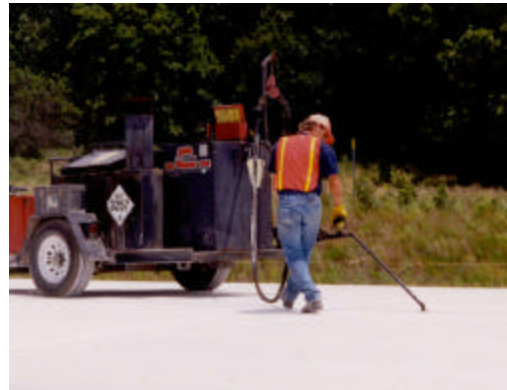
Figure 5. Installing Longitudinal Joint Filler (Cutco)
