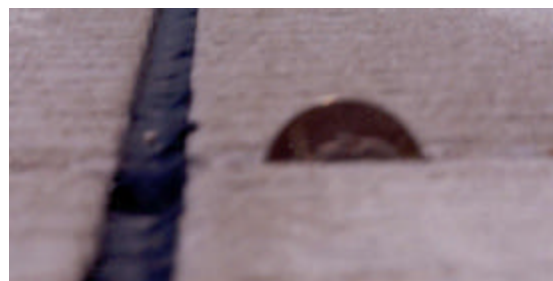
Figure 9. Joint Filler Installed in Longitudinal Joint Figure 10. Quarter Showing Depth of Backer Rod Before Sealing
