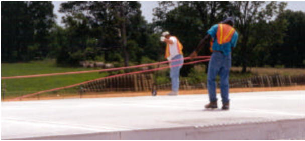
Figure 4. Placing Backer Rod (Cutco)
