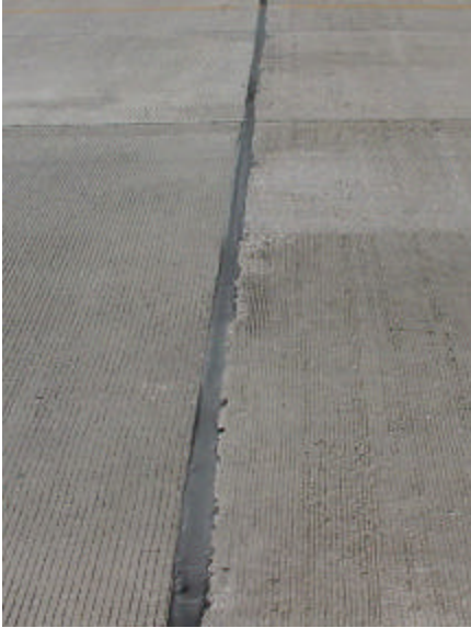
Figure 16. Conventional Joint Seal Method, RT 71
