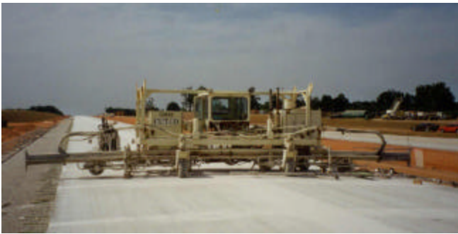
Figure 2. Longitudinal Sawing by Cutco
