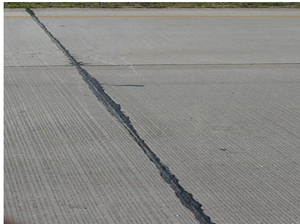
Figure 15. Conventional Joint Seal Method, RT 71
