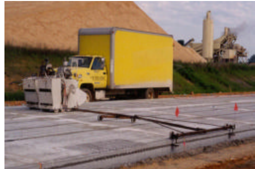
Figure 3. Transverse Sawing by Cutco
