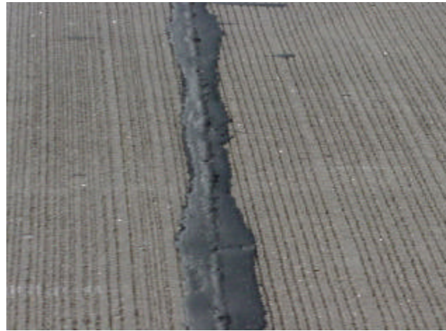
Figure 17. Conventional Joint Seal Method, RT 71
