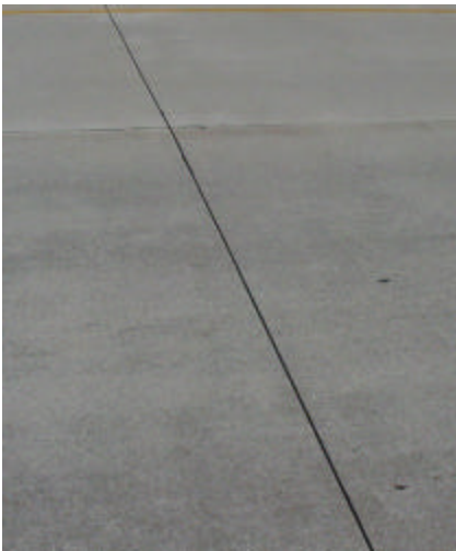
Figure 14. Cutco Joint Seal Method, RT 71
