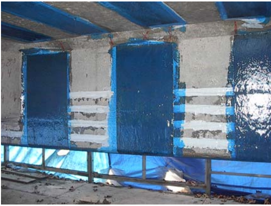
Figure 3 – Manual lay-up FRP Laminates
