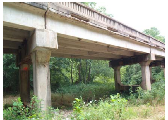
Figure 2 - Bridge T-0530 Crawford County
