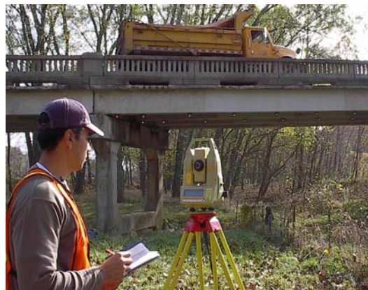
Figure 9 – H2O MoDOT Dump Trucks, Total Station and Mounted Prisms during Load Testing
