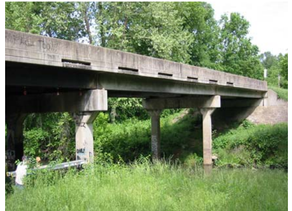
Figure 1 - Bridge P-0962 Dallas County
