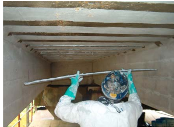
Figure 5 – Adhered Pre-Cured FRP Laminates
