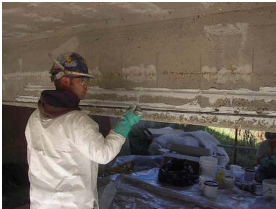
Figure 4 – Near Surface Mounted FRP Bars
