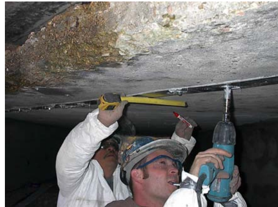
Figure 6 – Mechanically Fastened FRP Laminates
