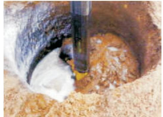
*Figure 1. Application of polymer-based drilling fluid (PDSCo, El Dorado, Arkansas).*
