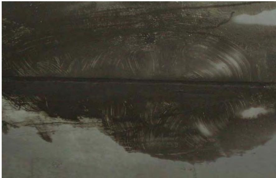
Figure 6 - Close up shows no cracking. Curing compound allowed on this job, but it should be noted that it was done in very mild October weather and was not exposed to sun as it was inside a tunnel.
