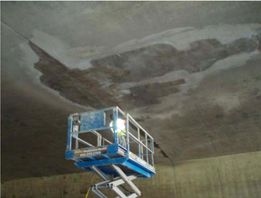
Figure 5 - Repairs on the underside joint of the roof of a tunnel bridge on Project J4I1699, NB I-35 in Kansas City. The dry method using pre-bagged mix did a good job here.
