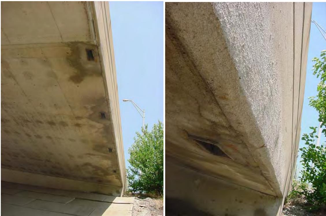
Figure 1 - Br. A2175, shotcrete patches around drains now 8 years old.
