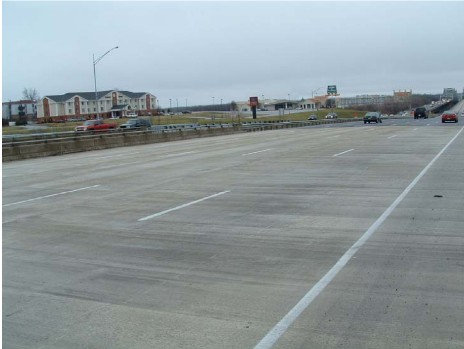
Figure 4: Finished LMC-VE overlay on Bridge No. A3582, the placement observed (inside shoulder and 1 ½ lanes) is in the foreground.
