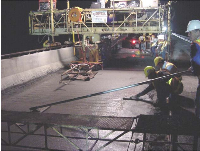
Figure 2: Last placement on Bridge No. A3582 - minimum finishing required.
