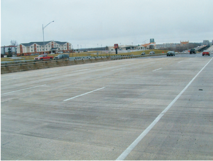
Figure 2 - LMC-VE overlays open to traffic on I-70, St. Charles County
