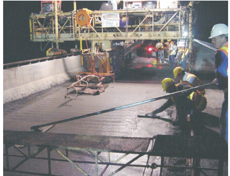
Figure 1 - Night operation on I-70, St. Charles County
