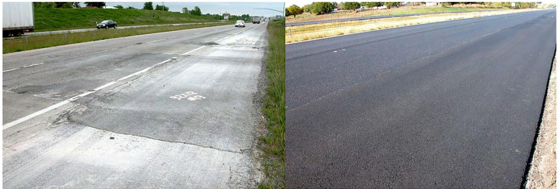
*Figure 1, Interstate 70 Pavements Before and After Pavement Resurfacing.*
