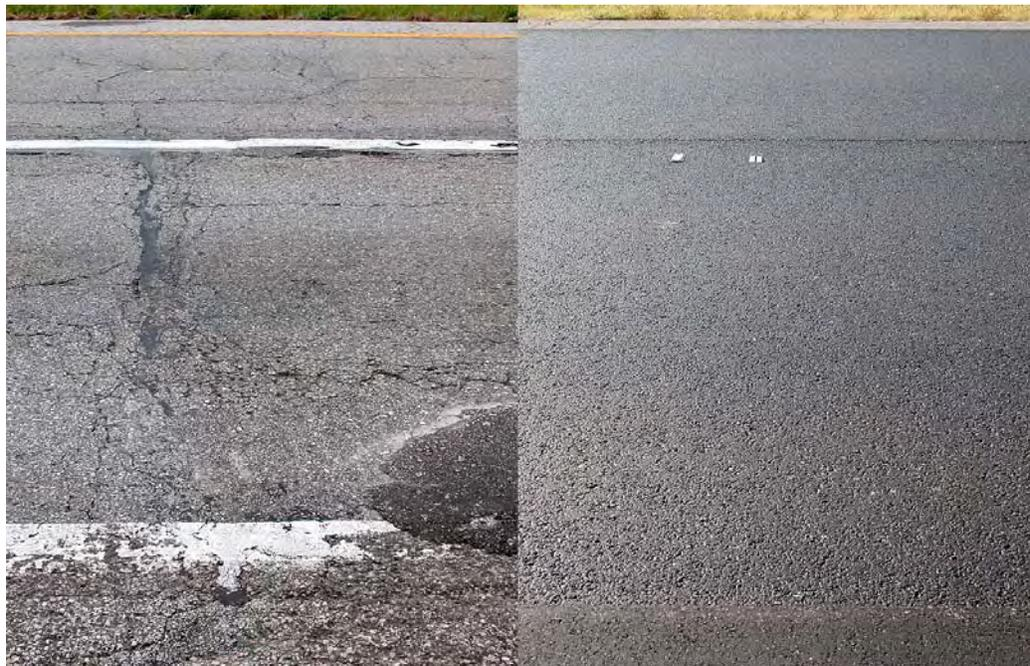
*Figure 4, Close-up of Pavements Before and After Resurfacing.*
