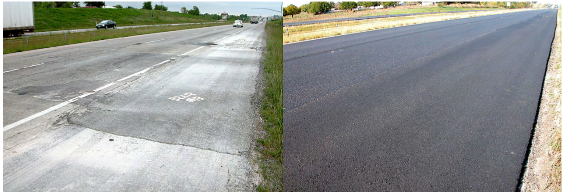
Figure 1, Interstate 70 Pavements Before and After Pavement Resurfacing.
