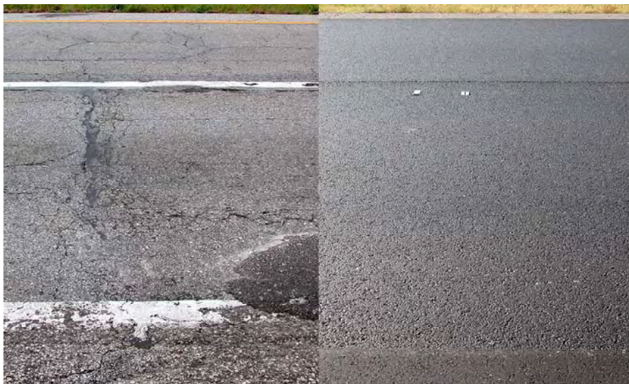
Figure 4, Close-up of Pavements Before and After Resurfacing.
