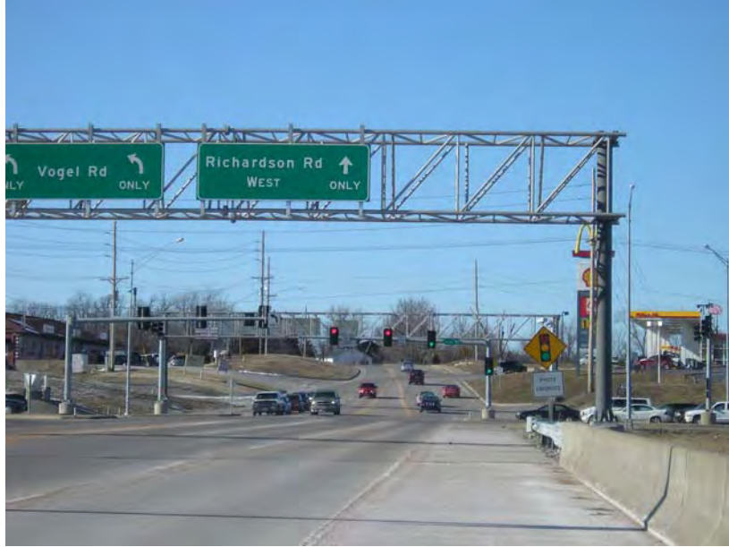
Figure 7: Intersection 3, Richardson Road at Vogel/I-55 with the Current Signs
