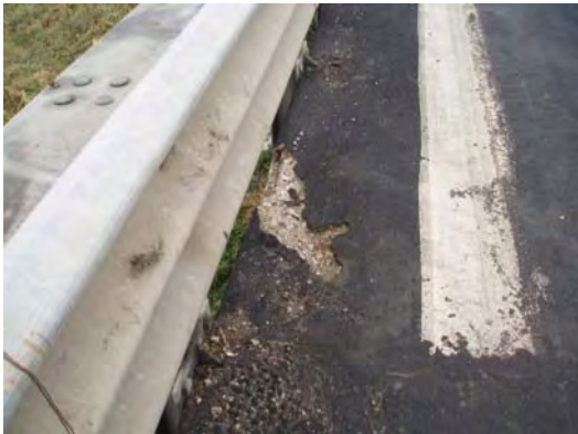
Spalling/loose areas
