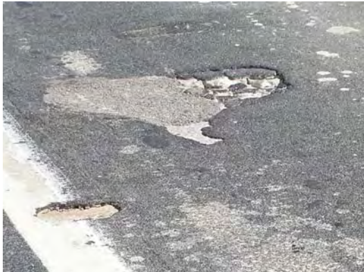
Sunken/cracked areas
