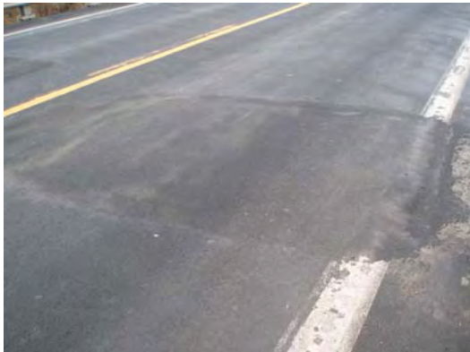
Post overlay Patches
