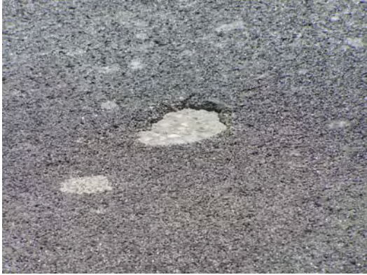
Delamination
