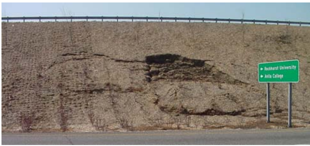
Figure 2. Typical surficial, or “nuisance” slide, appropriate for stabilization using recycled plastic reinforcement
