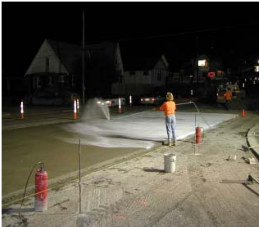
Application of the curing compound.
