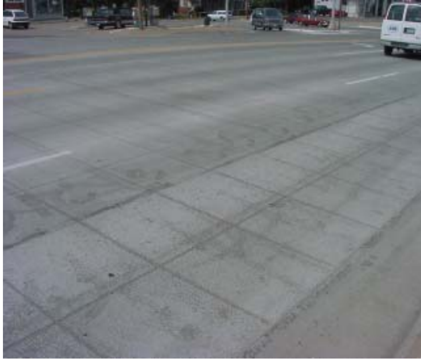
View of the 3-foot by 3-foot joint pattern.
