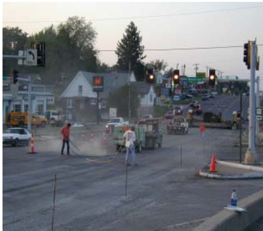
Contractor cleaning milled asphalt surface of debris using high-pressure air.
