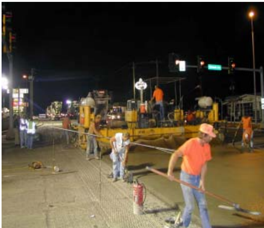
Contractor finishing fresh concrete behind paver.
