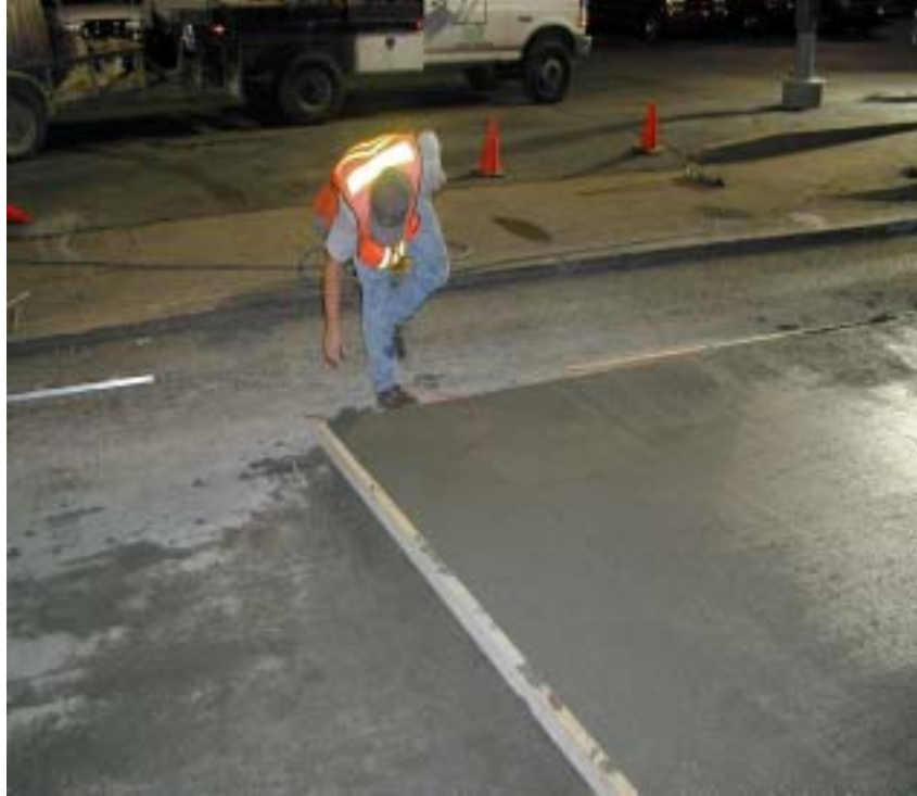
MoDOT Research Technician inserting thermocouple probe for maturity testing.
