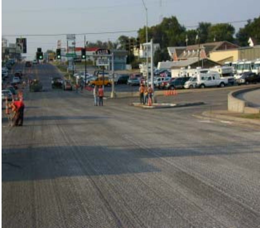
Texture of milled asphalt surface prior to concrete overlay placement.
