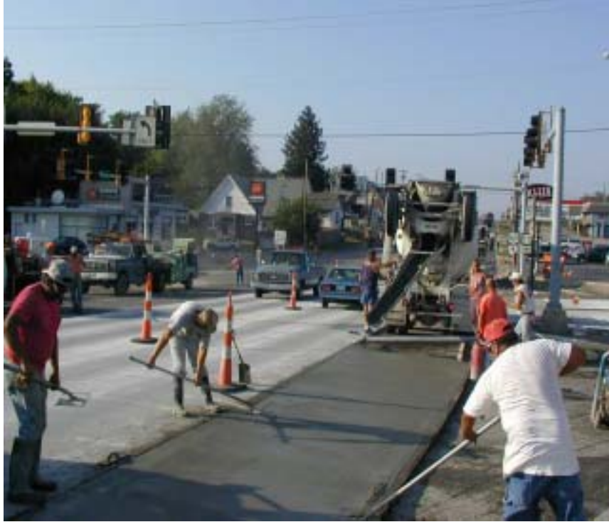
Contractor hand pouring a turn lane.
