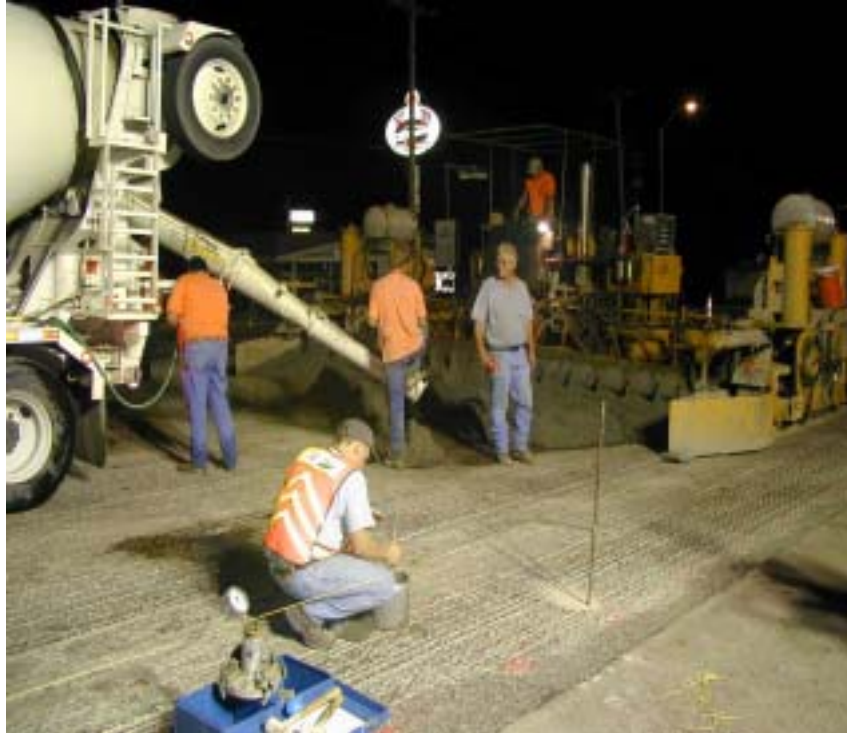
MoDOT Research Technician performing ASTM C231, air content of fresh concrete.
