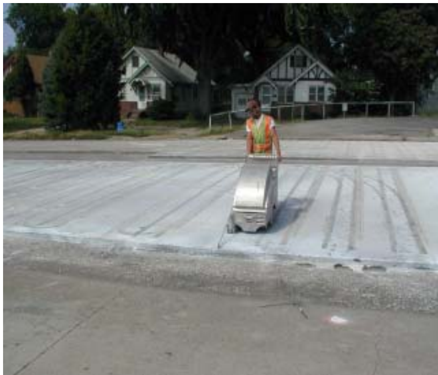
Early entry saws used on this project.
