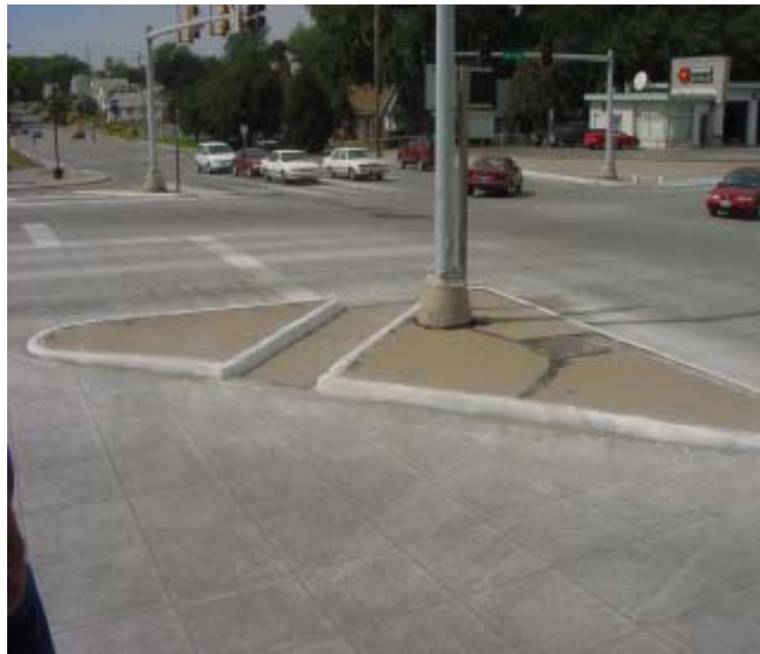
View showing the continuation of the joint pattern in the turn lane.
