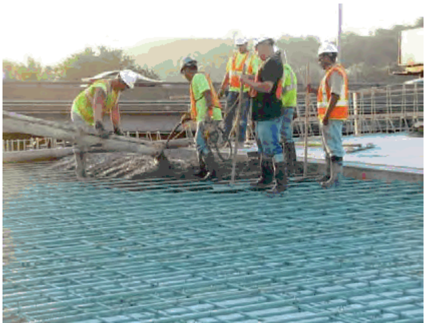
Pouring a bridge approach slab
