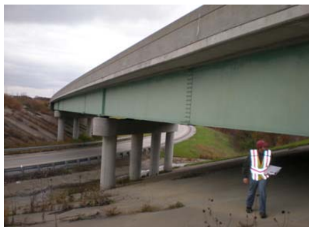
Field inspection of existing bridge coatings
