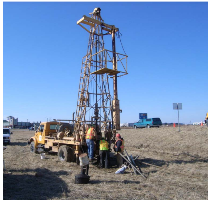
Drilling soil samples
