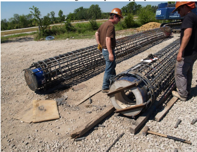
O-cell and rim cell attached to rebar cage
