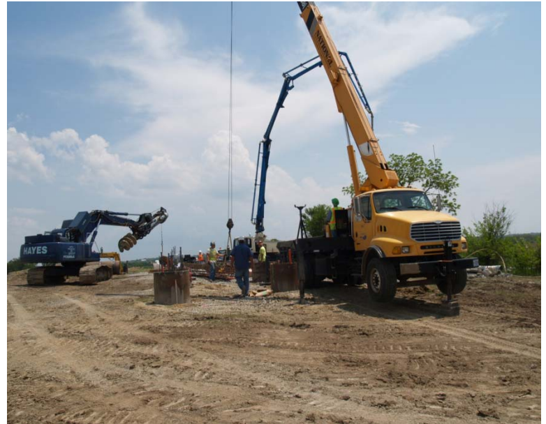
MoDOT boom truck and Hayes drill rig
