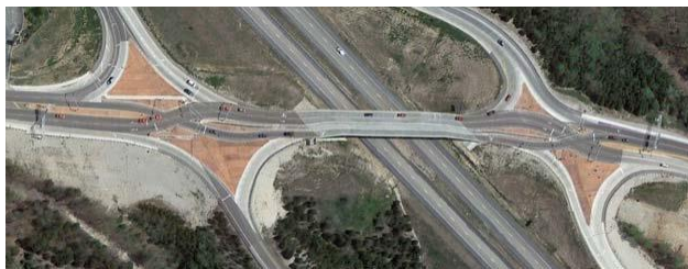
Aerial view of DDI at US 65 and MO 248, Branson, MO
