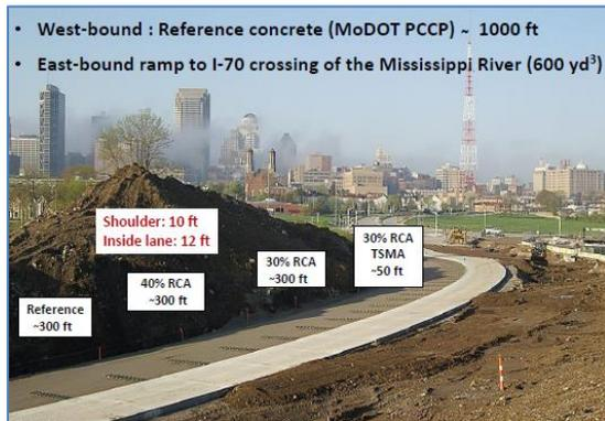
Researchers investigated the performance of three mixture proportions of concrete with varying amounts of RCA, water-to-cementitious materials ratios (w/cm), and Class C fly ash contents, as compared with a reference sample in order to develop a sustainable concrete
