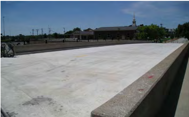
Completed Lafayette Bridge using LowP concrete.
